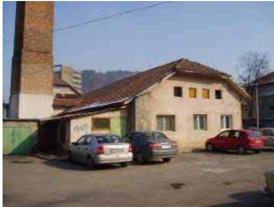
Figure 27: Old DH station with 6 x 0,5 MW gas boilers
