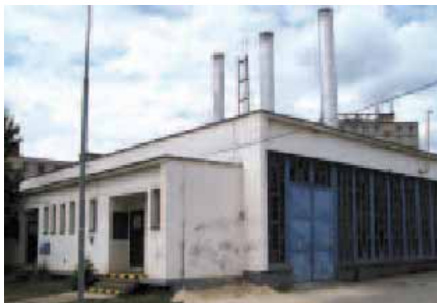
Figure 41: Outside-view of the boiler house
