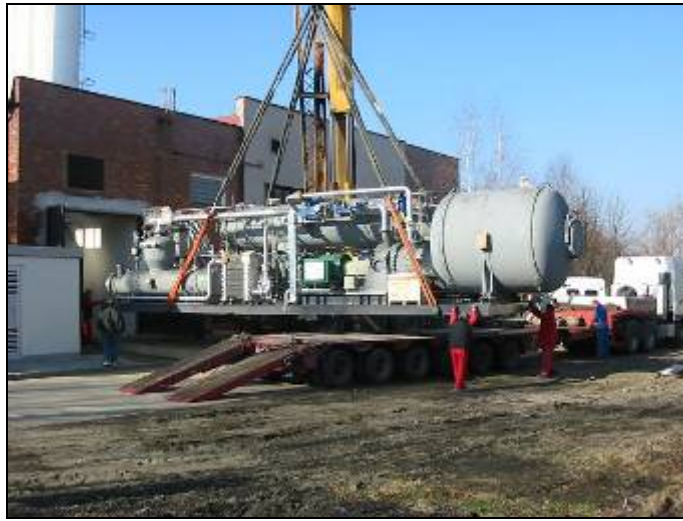
Figure 62: Trhové Sviny CHP plant – construction of the ORC module
