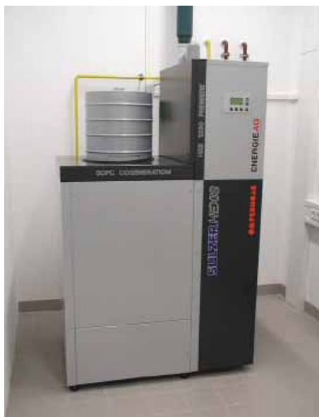
Figure 7 1 kW el SOFC system of Sulzer Hexis AG (Source: Energie AG)
