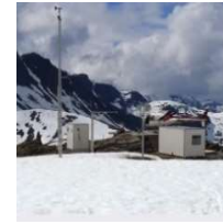
Backup power with Fronius H2 fuel cell
